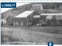
workshop and store. The generators in this building were powered by gas engines using gas produced on site from coal brought from Portreath harbour.
